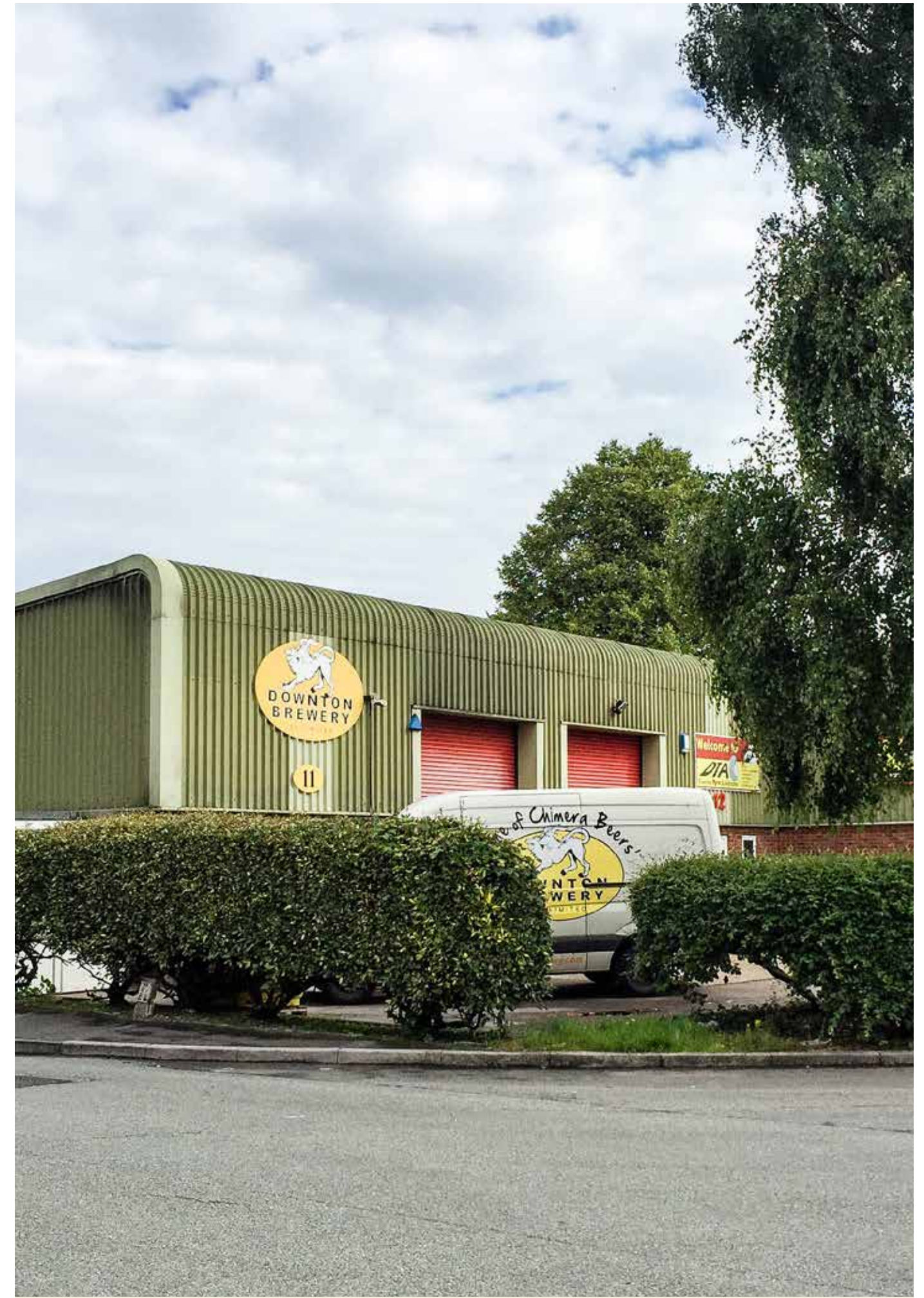
Units at Downton Business Park
